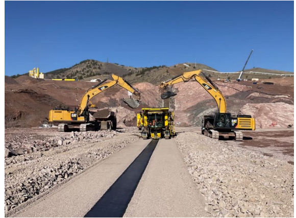
Chimney Hollow asphalt core construction
